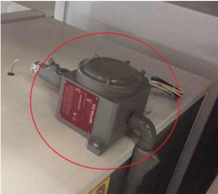
Mechanical Temperature Controller – located in the rear top location of refrigerator or freezer, inside of the metal enclosure.
